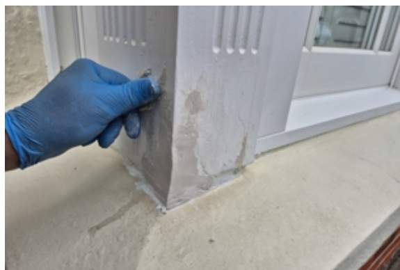
After rotted wood had been removed and the frame stabilised, AB Original filled all gaps in the corner
