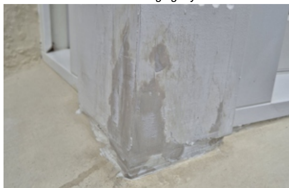
Once AB Original cured, it left the corner fully rebuilt
