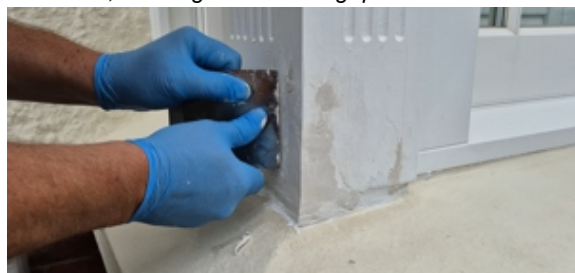
AB Original was smoothed off using a metal spreader and a little water before being lightly sanded down
