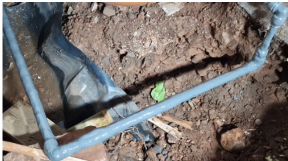
After surface damage was repaired with Superfast Aqua PW, the line was refurbished with Liquid Metal
