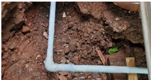
SylWrap HD provided an impact resistant sleeve to prevent stones damaging the pipe after reburial
