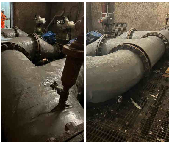
Liquid Metal and SylWrap Bandage combined to form a robust outer shield protecting against corrosion
