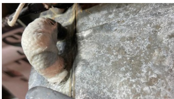
SylWrap HD forced the putty into the crack, creating a watertight seal and offering protection from future expansion of the pipe
