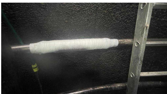
SylWrap HD encompassed the repair with a rock hard shield to protect against future impact from the pillar and mixer blade
