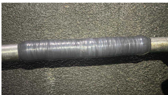
Wrap & Seal was applied along the entire 600mm length of the area which had been patch welded
