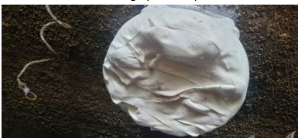
Completed repair with the entire stub encapsulated
