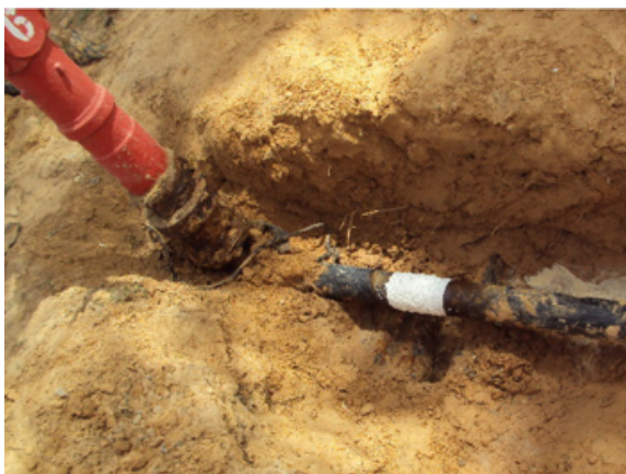
A trench was dug with enough clearance to reach the below-ground section of pipe, which was then repaired using Wrap & Seal and SylWrap HD
