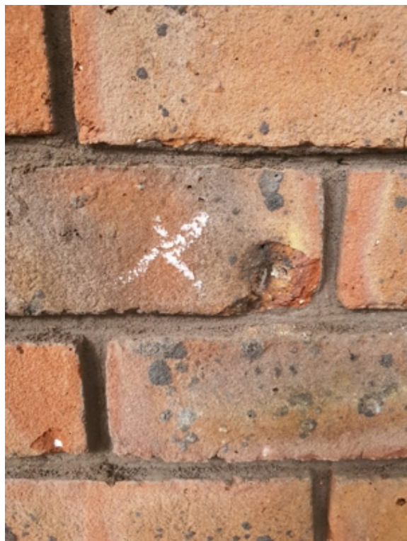
Damaged caused by lime blow can be seen next to the 'X' marked in the brickwork
