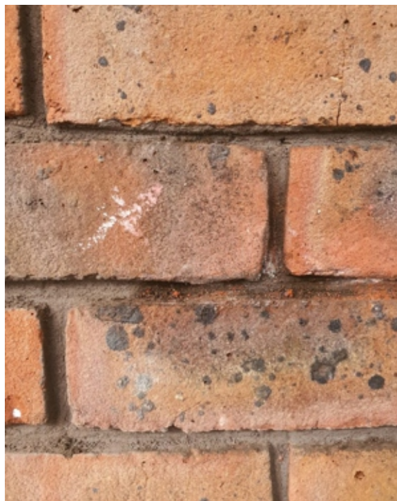
AB Original mixed with brick dust and then spittled with a wire brush created a seamless repair
