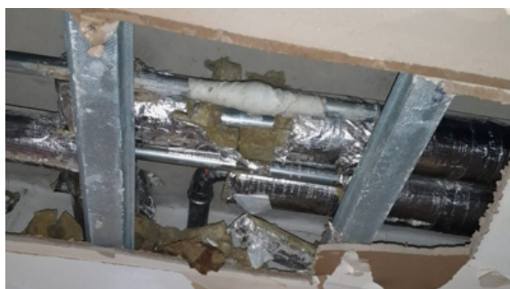
SylWrap HD encapsulated the pipe to finish the repair
