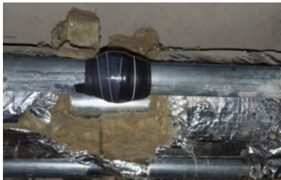
Wrap & Seal applied to seal all leak areas
