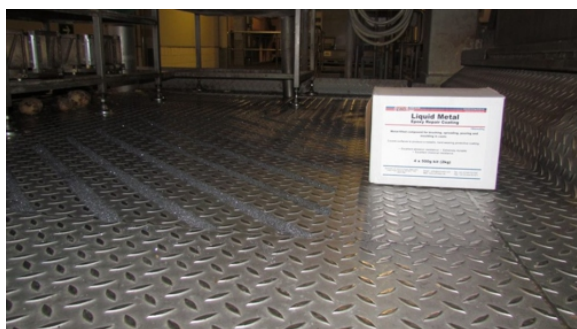
Liquid Metal was painted onto the surface in strips marked with masking tape and silicone carbide grit sprinkled on top
