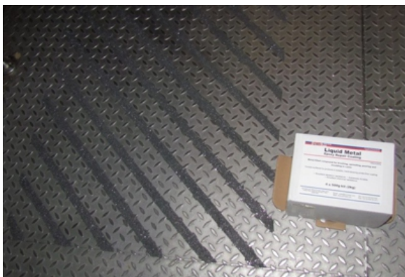
Once cured, Liquid Metal permanently bonded the grit to the flooring, creating an anti slip surface
