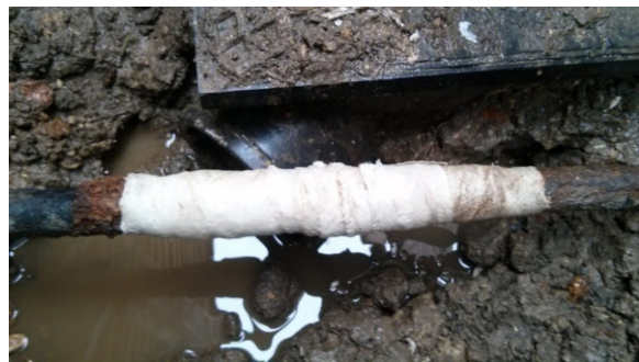
Completed repair wrapped in a SylWrap HD Pipe Repair Bandage before being re-buried
