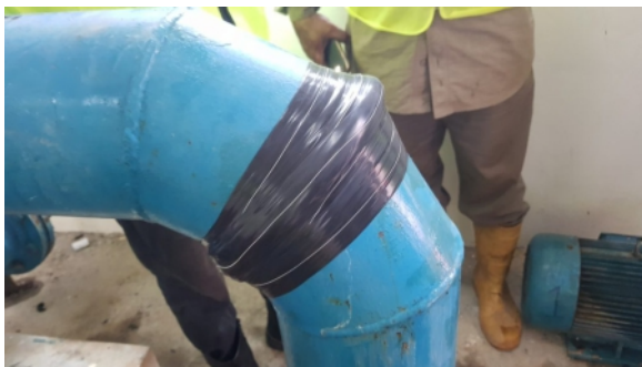
Wrap & Seal was stretched by 300 percent, fusing to form a solid silicone band over the pinhole
