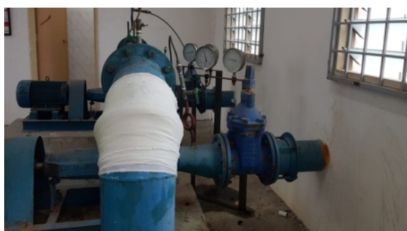
The repair of the elbow was completed in under 30 minutes with no disruption to the pumping station
