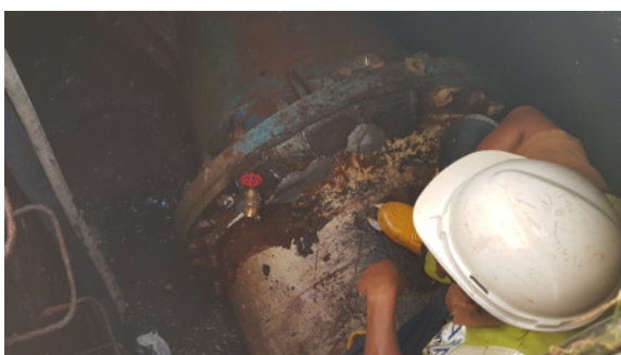
The 'impossible' repair completed with a tap fitted
