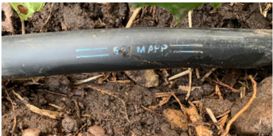
The hose had been badly cut by a pruning saw
