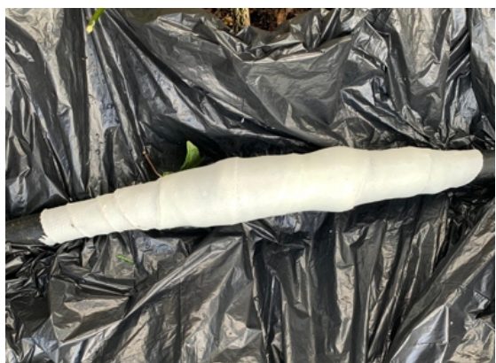
Completed repair with SylWrap HD applied to cover the entire damage area
