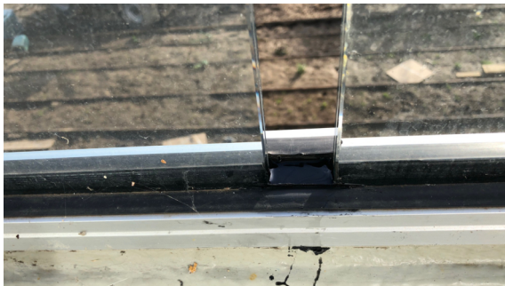
Liquid Rubber poured into the gap as a filler
