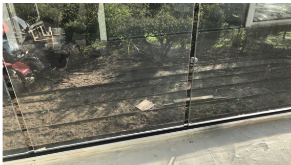
The completed repair sealed the gaps to prevent damage occurring to the electrical equipment below
