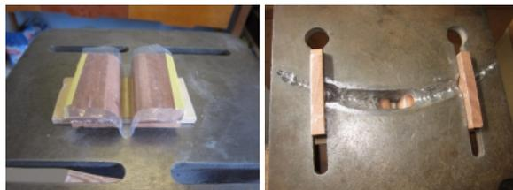
Wood used to prevent epoxy paste from passing through the gouge or curing in gaps in the base
