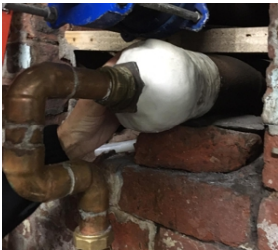
The completed repair with the pipe encompassed with Sylmasta AB Original
