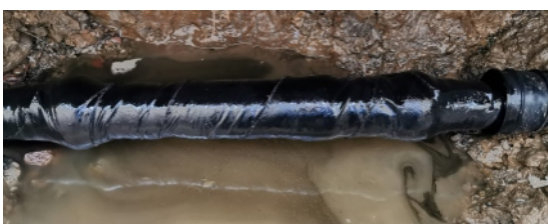
Second SylWrap HD Bandage encompassed entire pipe, painted black to appear uniform
