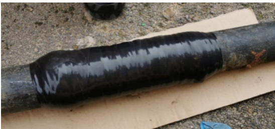
Wrap & Seal increased the pressure resistance
