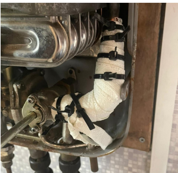
Space constraints meant SylWrap HD was cable tied in place whilst it cured to reinforce the pipe
