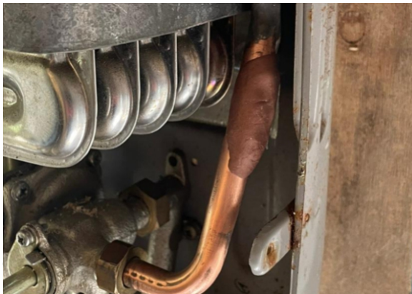
Superfast Copper plugged the hole in the pipe
