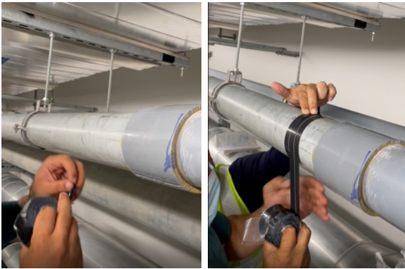
The pipe was leaking from the left hand side of the joint with the application of Wrap & Seal starting 100mm away to build up a ridge towards the step
