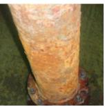
Lower sections of the pipe were badly corroded
