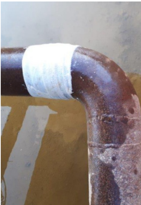
Superfast Steel was used to plug the pinhole. The repair was then reinforced with SylWrap HD, which provided it with a rock-hard, impact resistant protective sleeve
