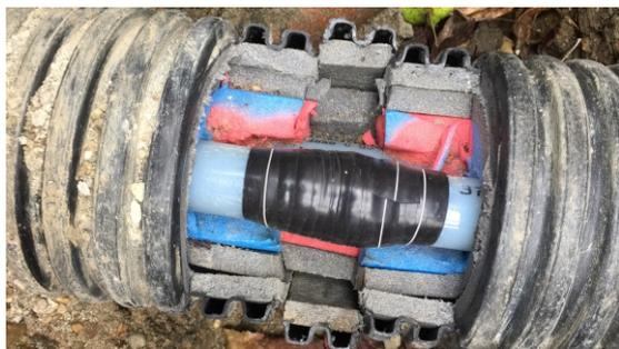
The heating pipe repaired with Wrap & Seal after the outer pipe and insulation lagging were cut away
