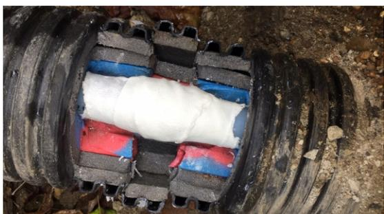
SylWrap HD added a further layer of protection to the pipe from the farm's building works
