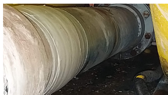
Further SylWrap was then applied to the pipe to strengthen and protect it from future wear and tear
