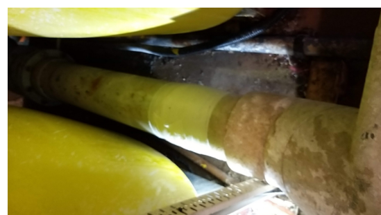
SylWrap HD Pipe Repair Bandage provided an impact resistant layer over the initial repair
