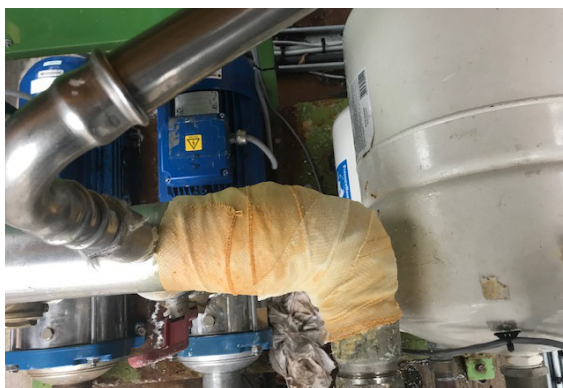
SylWrap HD provided an impact resistant layer over the initial repair. It tinged red because of the high temperature but could be painted to match the pipe at a later date if required
